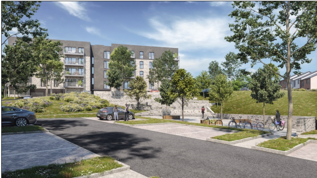
Figure 3.11: CGI of the central area of 'Option A', showing the substantial use of retaining Walls to address the 3m level change.
